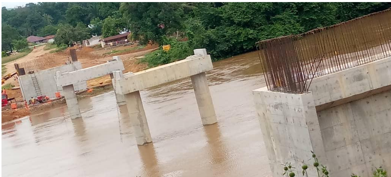
Ongoing construction of the Tomparie bridge
