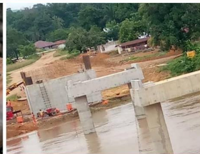
Constructing four rural bridges in Tomparie, Manowa, Mattru, and Gendema.
